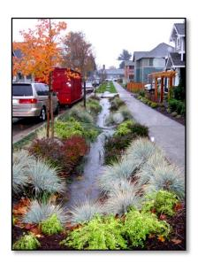
D. Bioswales or Retention Ponds: Bioswales and Retention ponds are vegetated landscaped depressions that capture, treat, and slow down stormwater runoff. They provide opportunities to treat stormwater on-site and are a more aesthetically pleasing environment than the typical required concrete stormwater fixtures.
